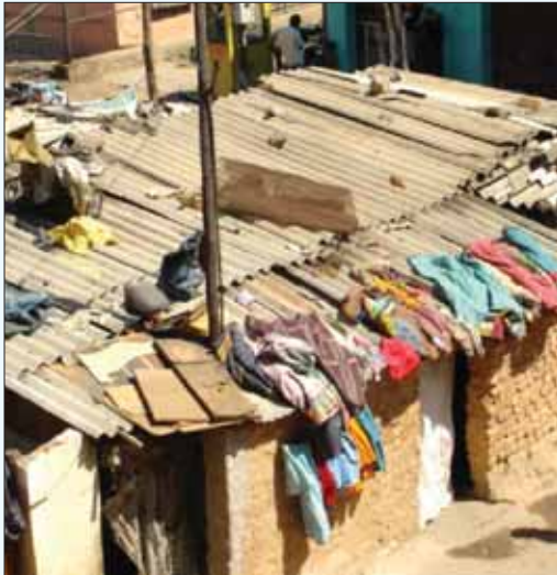
Typical AC roofing in New Lingarajapuram, Bangalore. Note lack of ventilation apart from that available by using the doorway.
