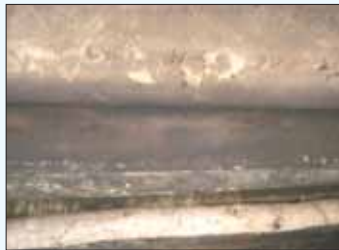
Flaking and pitted AC roofing, resulting from smoke damage. House was newly built and had been occupied for one year at the time of survey.
