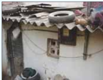
Typical exterior condition of AC roofing in New Lingarajapuram. Note the broken AC roofing sheets, low roof height and the ventilation 'window'—a typical size in the homes of New Lingarajapuram.
