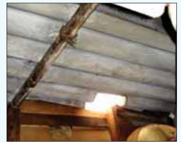
Homemade skylight cut into AC roofing, the cutting of which releases harmful chrysotile fibres into the environment. The roof has been previously painted with white emulsion paint which deteriorates rapidly, often showing signs of discolouration and mould. Note the contrast in ceiling colour when compared to white ceiling fan (top right).
